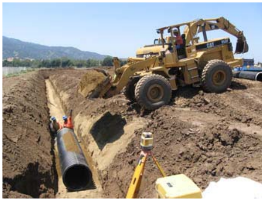
Site storm drainage installation has started!
