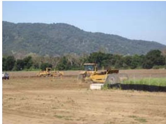
Site grading has started!
