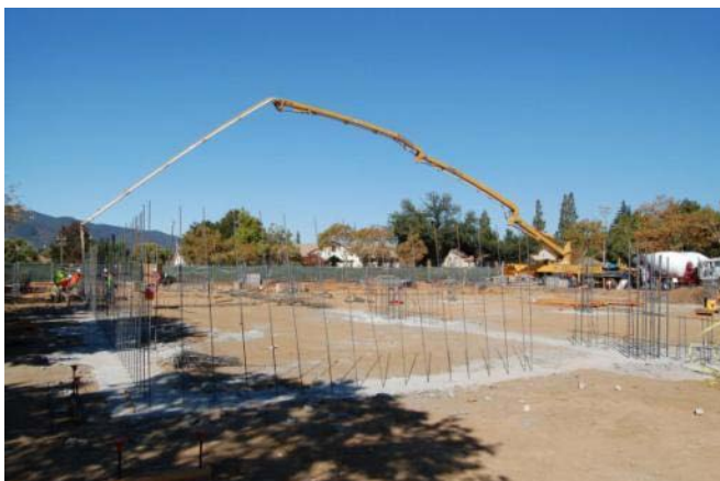
Concrete being pumped into the foundation
