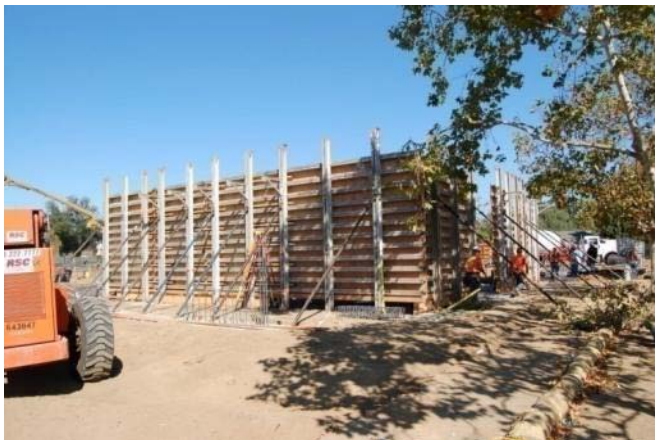
Forms for poured in place concrete walls are erected
