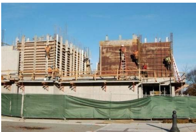
Workers forming walls at South west corner of building
