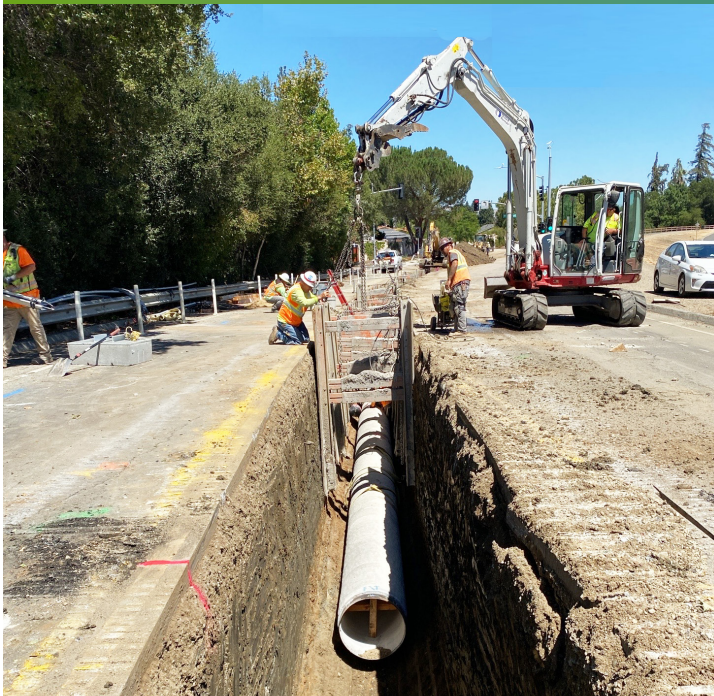
Crews installing the recycled water pipeline along W. Luchessa Ave.
